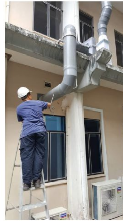
Fume Hood & Local Exhaust Ventilation Installation, Universiti Teknologi Malaysia
