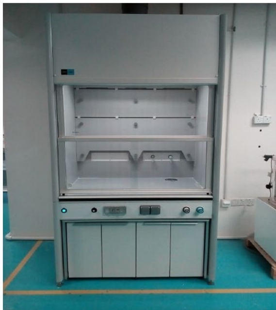
Fume Hood & Local Exhaust Ventilation Installation, Universiti Malaysia Perlis
